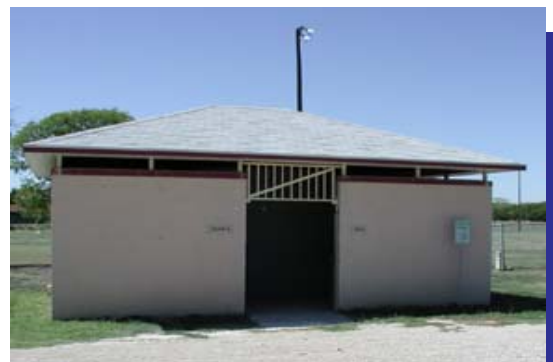
Restroom facilities at Salmon Park will be renovated.
