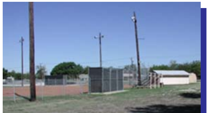
Ball fields, lighting and fencing will be upgraded.
